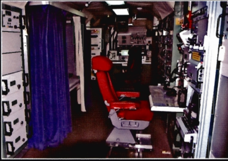
Left: Underground launch control center at Delta-01.
