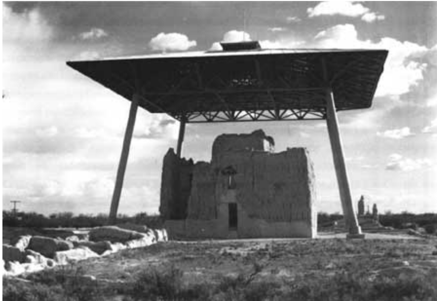
Figure 22: The 1932 Ruin Shelter Roof Courtesy of the Western Archeological and Conservation Center
