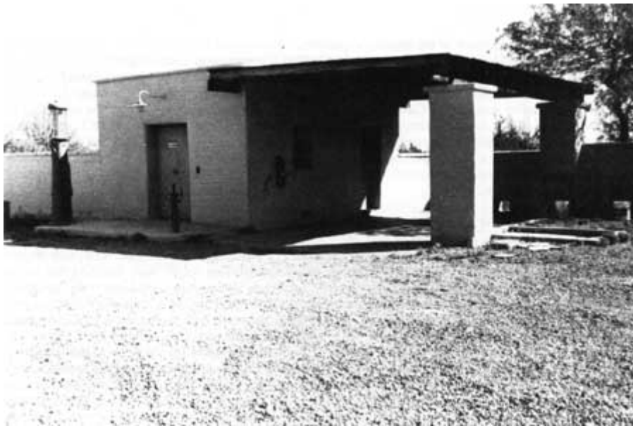
Figure 41: Building 8 — Oil house with wash rack.
