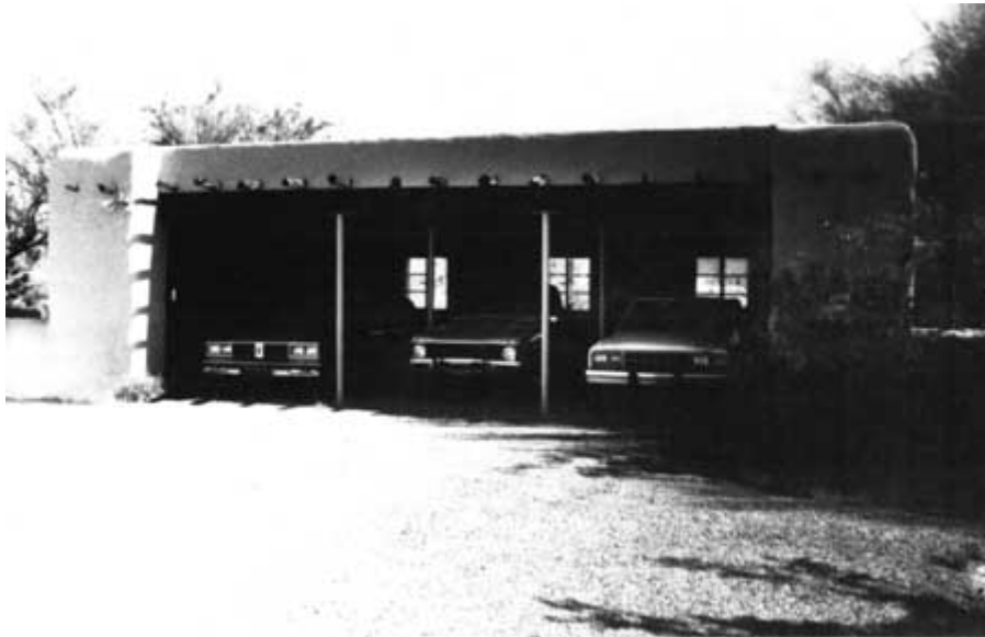
Figure 38: Building 15 — Originally a tool and implement shed when it was built in 1931. It became a laundry in 1940 and was modified to a three car garage in 1963.
