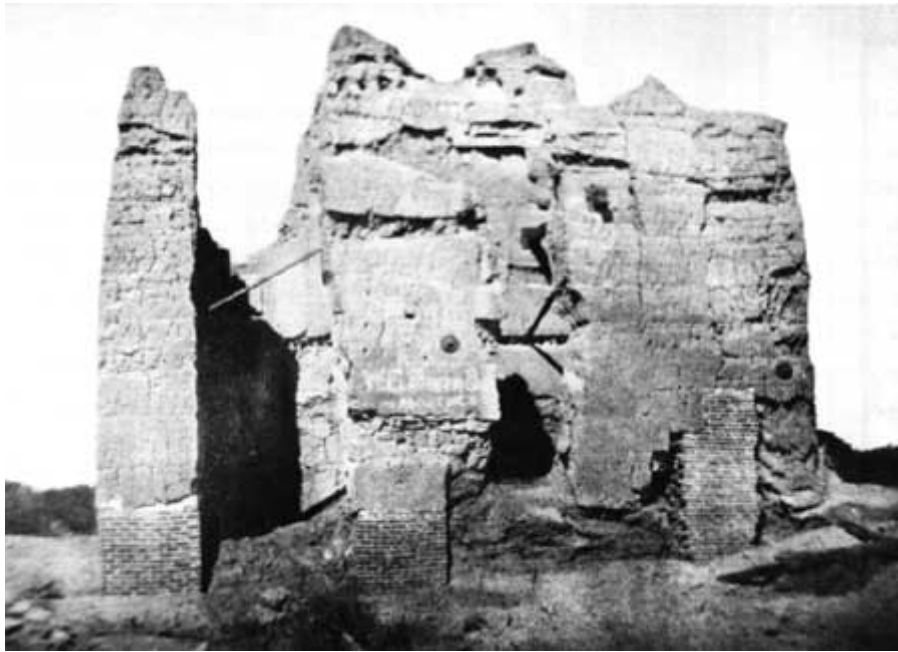
Figure 9: The Great House Viewed from the South 1891 This photograph shows the brick work before it was faced with concrete Courtesy of Casa Grande Ruins National Monument
