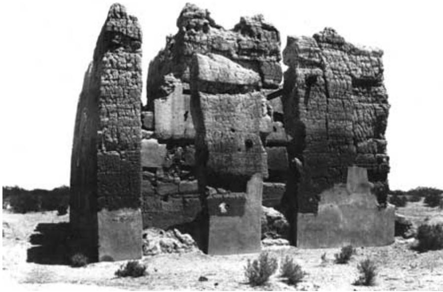
Figure 10: The Casa Grande Viewed from the South Ca. 1902. This photograph shows the concrete facing on the brick. Courtesy of the Colorado Historical Society.
