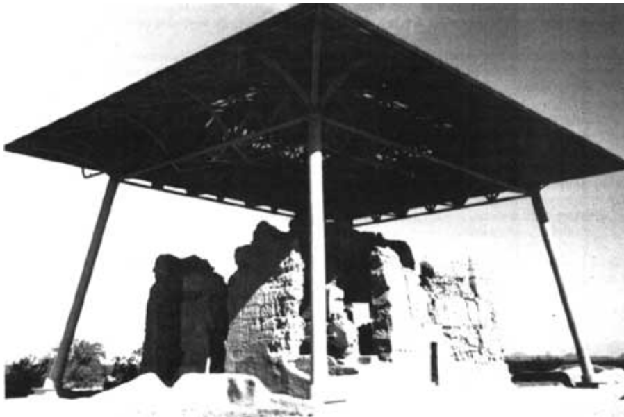
Figure 50: Ruin Shelter Roof. Constructed in 1932 to protect the Great House.
