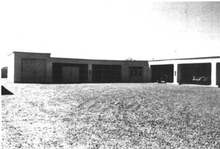
Figure 44: Building 10 — An L-shaped equipment storage building.
