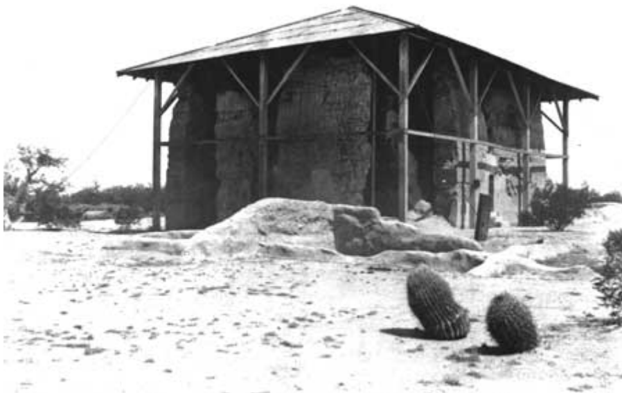
Figure 14: The First Ruins Shelter Roof Constructed in 1903. This ca. 1925 photograph shows the anchor cables that provided stability. Courtesy of the Western Archeological and Conservation Center.
