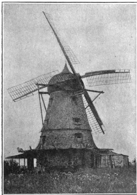
The "Old Mill" at Lawrence, erected in 1863. This was a gristmill, an octagon shaped, four-story structure, having a genuine Holland windmill for motive power. Additional buildings were erected for the manufacture of wagons and farming implements. The mill was abandoned many years ago, and in 1905 it burned.
